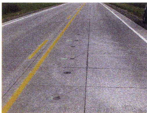
Figure 4-2 Temperature and Strain Gages Along Iowa Highway 13
